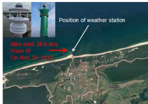
Fig. 2: Meteorological station in Leba (Polish N coast) is placed on top a lighthouse and consists of a SmartGuard logger, a GSM modem and a Gill GMX 600 weather sensor. A similar system is installed in Gdynia it is on-line and serves also for navigation aid.
